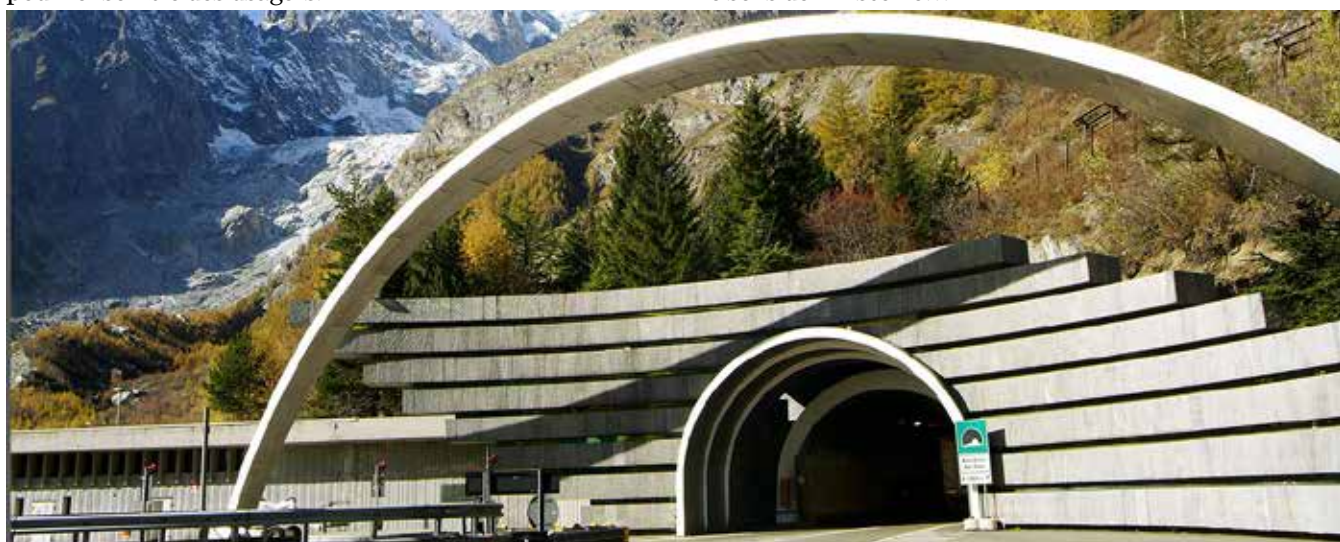
© Shutterstock - Tunnel Mont-Blanc
